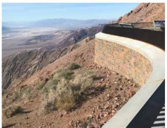
The approximately 5,000 square foot wall is designed in a serpentine shape, and includes two overlooks that jut over the hilltop. A thick cement cap and railing are mounted on top of the retaining wall to protect visitors. A large plaza for walking and parking was reconstructed and new seating was installed for the site. A tactile map made of bronze, designed by artist Bridget Keimel, was a new addition to the site's interpretive signage.
